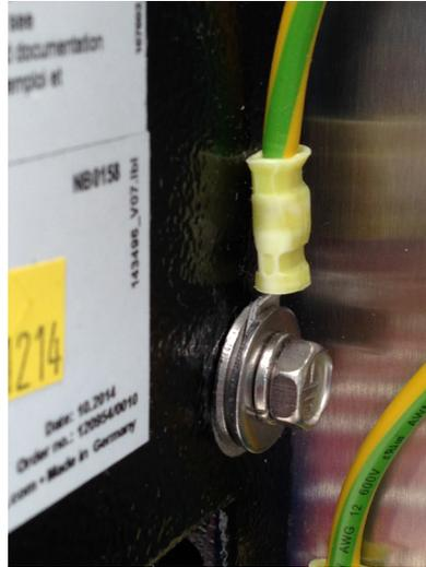
**Figure 4** *Earth Bolt and Nut Washer Assembly*
